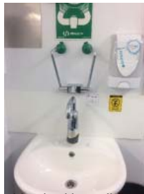
Splashback with no tile grout
