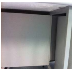
Under-bench pipes enclosed to prevent contamination and surfaces able to be cleaned/decontaminated
