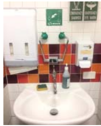
Splashbacks with absorbent tile grout
