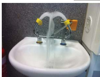
Correct installation and shorter length eyewash arm to allow water to drain into basin
