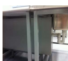
Under-bench pipes enclosed to prevent contamination and surfaces able to be cleaned/decontaminated
