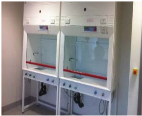
Fume cupboards with open top
