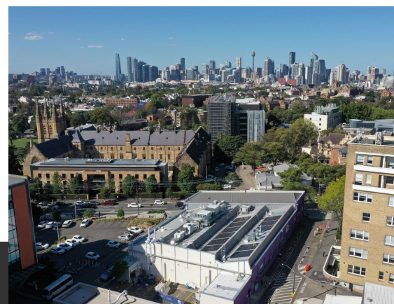
RPA Pathology, Sydney – Refurbishment
